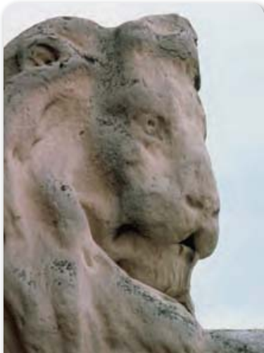
■ Figure 7.4 This statue has been chemically weathered by acidic water and atmospheric pollutants.
